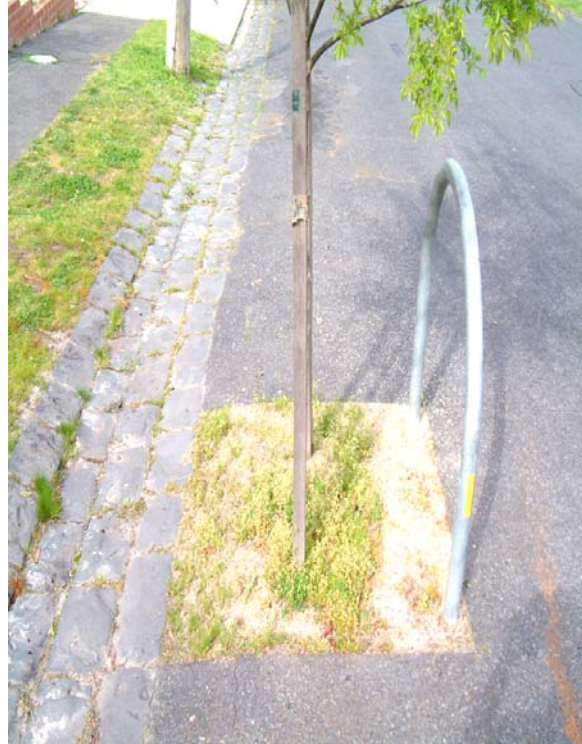
Close view emphasizes bitumen cut-out.
